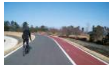
Construction of dedicated bicycle lanes
