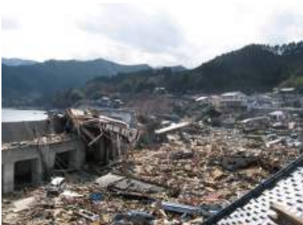
Tsunami Barrier devastated by the Great East Japan Earthquake
