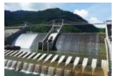
Water Supply (Potable)
