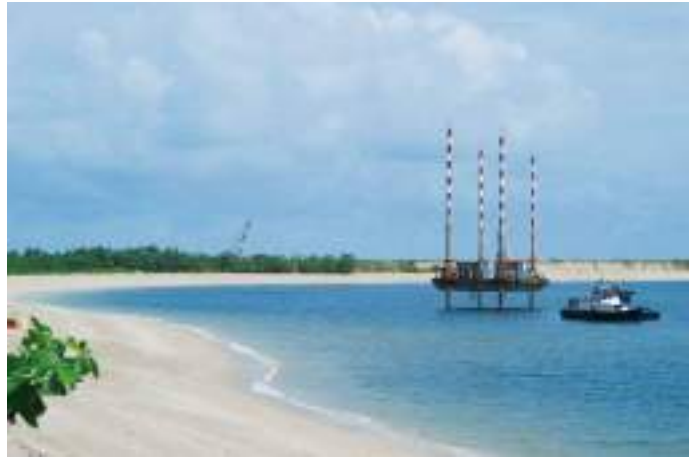
Off-shore Boring Survey on Jack-up Platform
