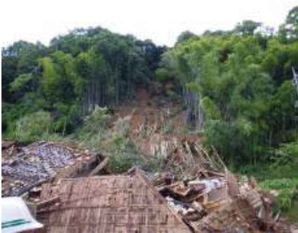
Damage from a Landslide
