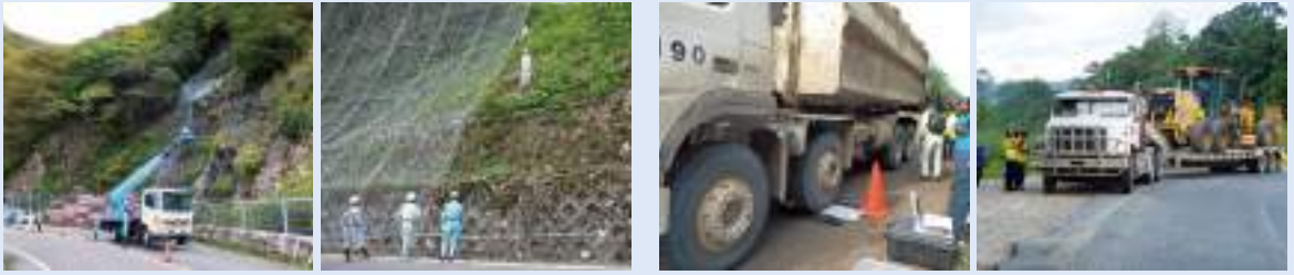
Inspection of cut slope
