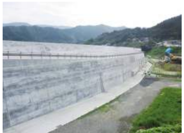
Restoration and Countermeasure Against Tsunami
