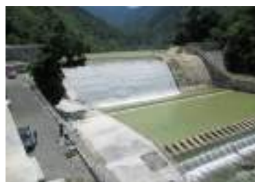
Small Hydro Plant
